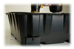
**Step 3:** Once positioned for final mounting, drill through dimples in four mounting bosses down through the C brackets.
